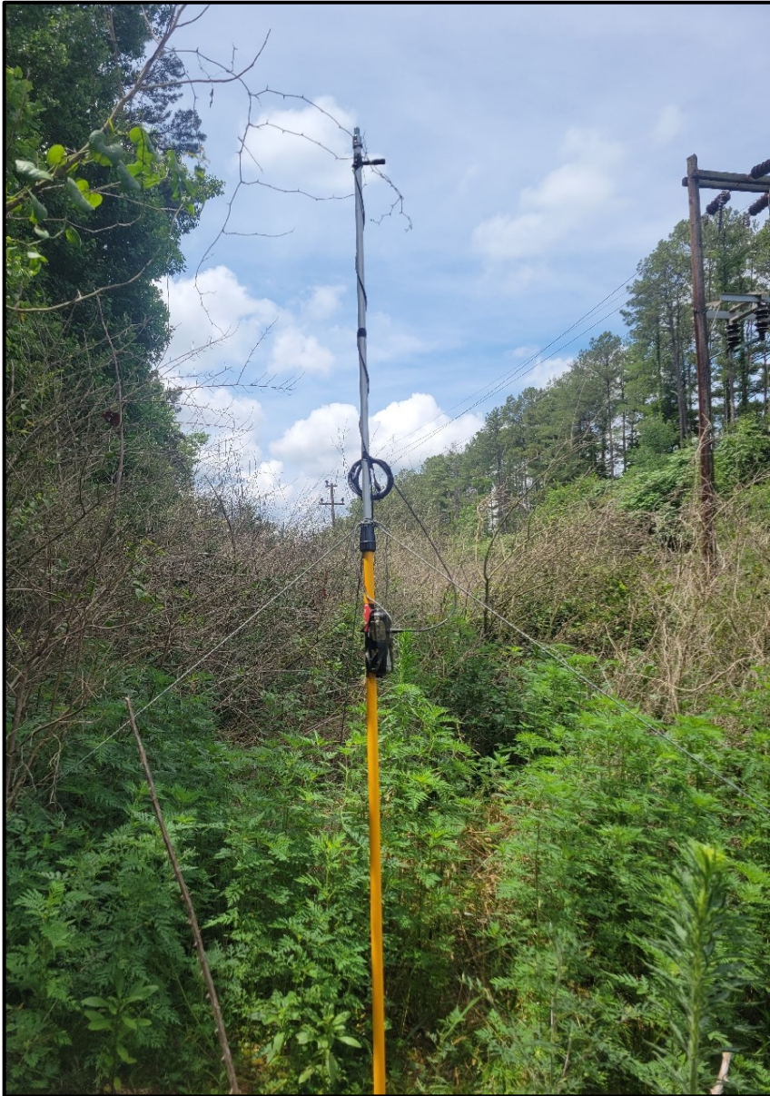
Photograph 9. KING 9, facing west (6/22/2022).
